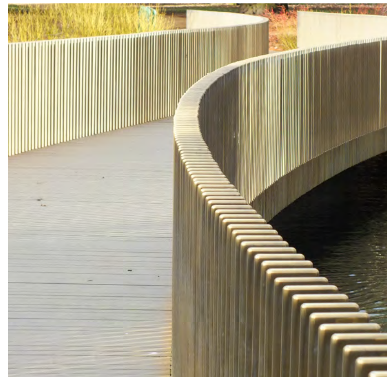
Metal vertical fins to provide security above masonry wall depth and spacing of fins will provide varying degrees of visibility into the school site which will change as viewers pass by responding to their angle of view
