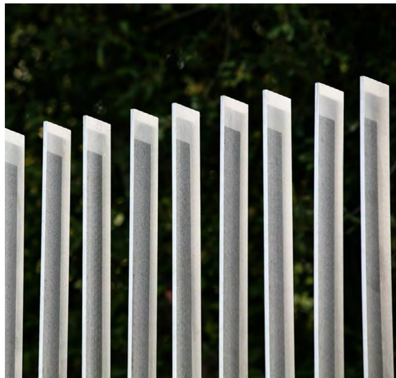
Metal vertical fins to provide security above masonry wall depth and spacing of fins will provide varying degrees of visibility into the school site which will change as viewers pass by responding to their angle of view
